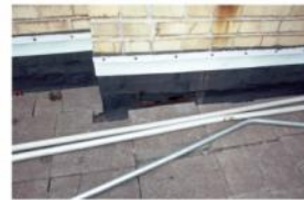
5th floor parapet. Repair condition using EPDM roofing and aluminum flashing (August 2004).
