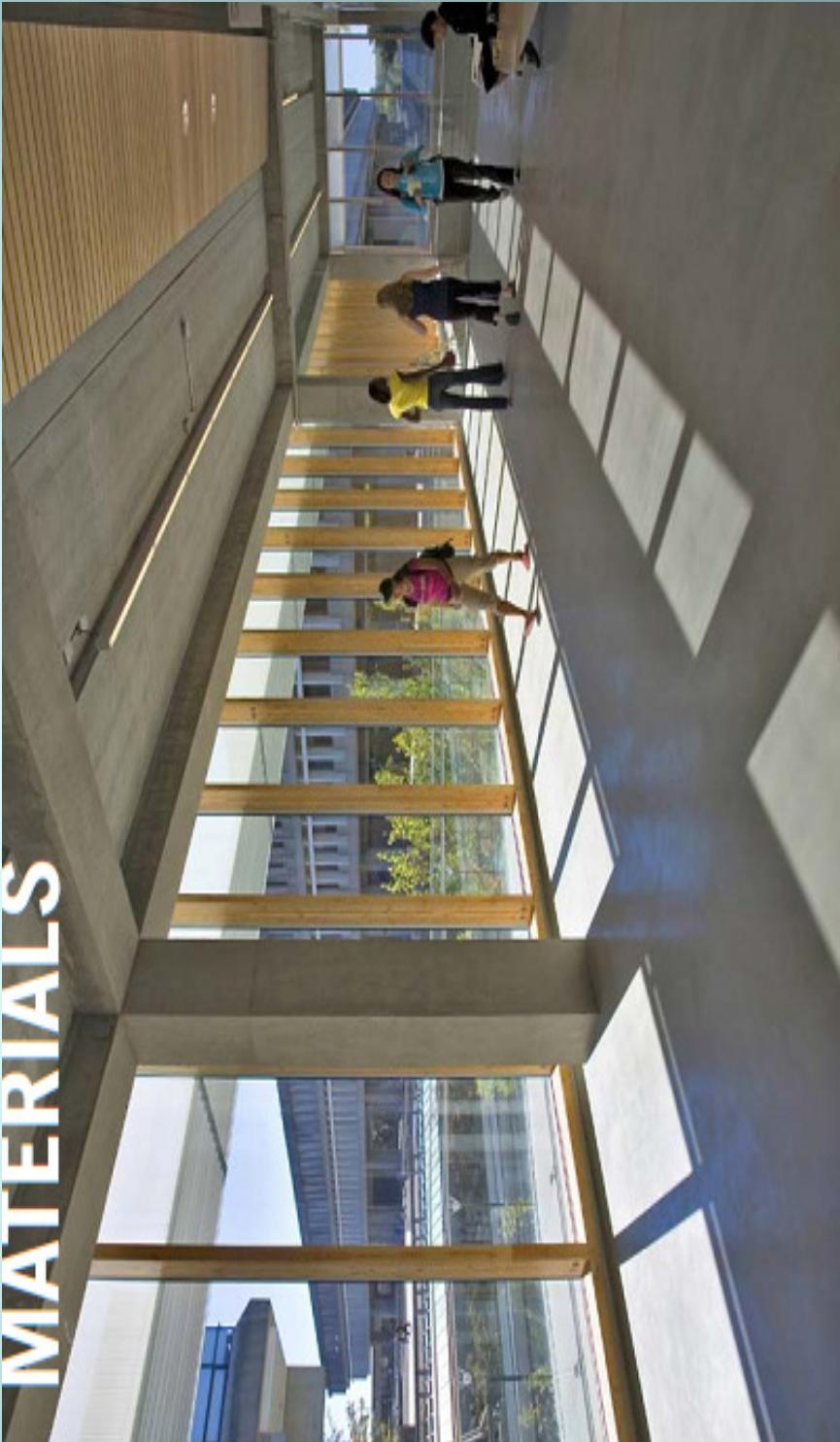
The materials in Blusson Hall were chosen for their beauty, durability and environmental properties. The exposed architectural concrete substitutes fly ash for 30-50% of the cement, thereby reducing the energy needed to make concrete and diverting a waste product from landfills. Fritted glass allows daylight through while reducing solar heat gain year round. Glulam window
