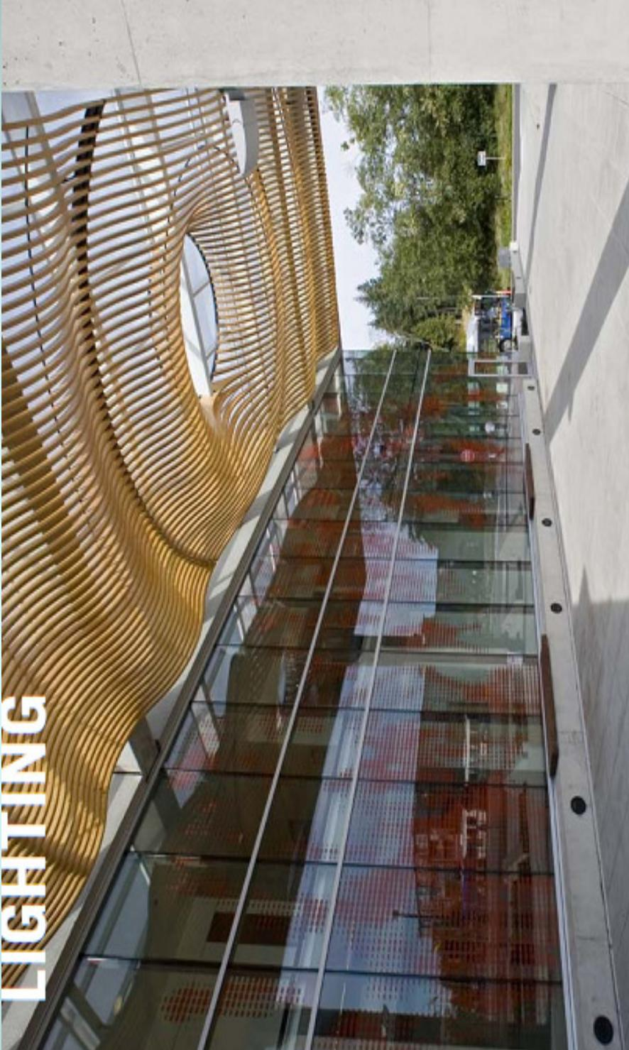
The design of Blusson Hall includes narrow floor plates that allow daylight into all areas of the building. Furthermore, each building elevation was extensively studied with Ecotect modeling software in order to develop the most effective solar strategy for each orientation, resulting in the use of horizontal, vertical, and angled sunshades depending up the sun's path.
