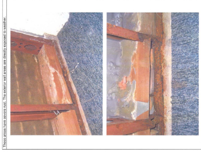
rusted sill plate - protected face
