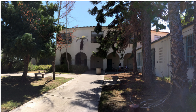
e view of existing courtyard
