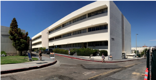
d view of existing engineering building
