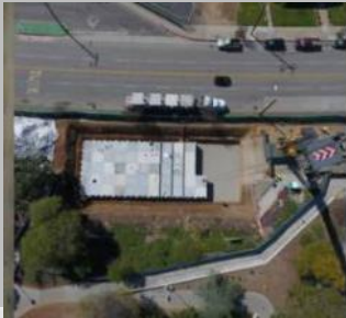
Buried Detention System at Mazeroski Field
