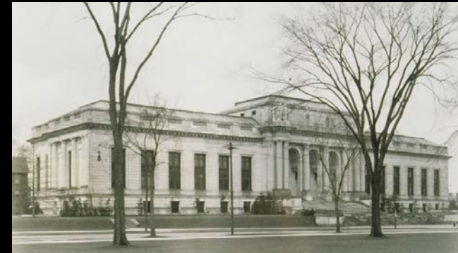
Connecticut State Library and Supreme Court Building (1910)
